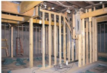
Figure 5. The new bathroom required a sewage ejector pump (left), which is located in the middle of one of the footings designed for the basement's bearing walls (above).
