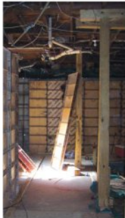
Figure 4. Pressure-treated 2x4s shot into the footing restrained the bottom of the one-sided wall forms (left); diagonal braces secured to temporary posts and the floor framing above held the top and middle (right).
