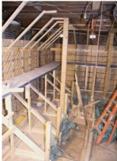
Figure 4. Pressure-treated 2x4s shot into the footing restrained the bottom of the one-sided wall forms (left); diagonal braces secured to temporary posts and the floor framing above held the top and middle (right).
