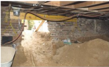
Figure 1. Because the home's tight lot lines limited access (top), all the excavation for the basement addition was done by hand, with dirt removed by wheelbarrow through a small opening in the foundation (above). The clay-shale soil was firm enough to allow for nearly vertical dirt walls within 2 feet of the existing brick footing (right).
