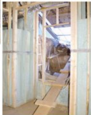
Figure 6. LVL beams now support the first floor, with room above for mechanicals (left). New stud walls around the perimeter were insulated with high-density polyurethane sprayed directly against the new concrete and existing brick (below left). The new space includes two egress windows (below right) and a large exercise and media room (bottom).
