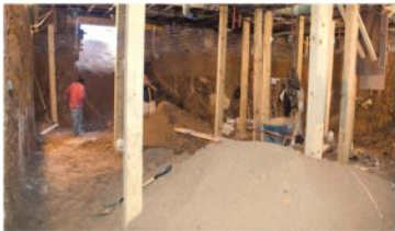
Figure 1. Because the home's tight lot lines limited access (top), all the excavation for the basement addition was done by hand, with dirt removed by wheelbarrow through a small opening in the foundation (above). The clay-shale soil was firm enough to allow for nearly vertical dirt walls within 2 feet of the existing brick footing (right).
